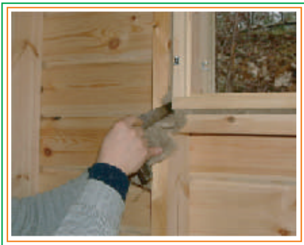
9. Check the sealing in the window corners.
