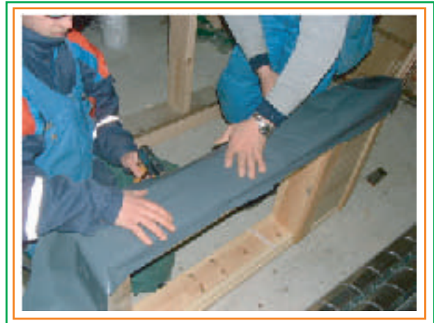
4. Tack one side of the plastic strip to the window frame, compress the ISOLINA flax insulation and tack the strip to the other side of the frame.
