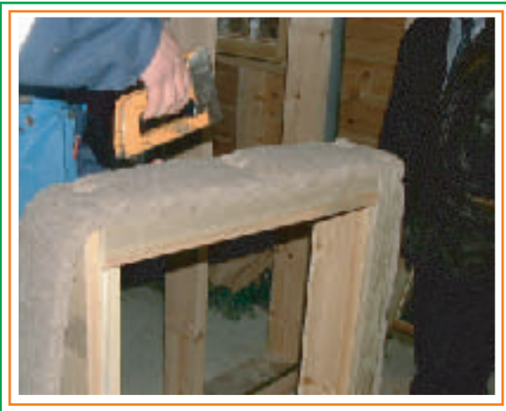
3. Fasten the ISOLINA flax insulation on the window frame with a tackers.
