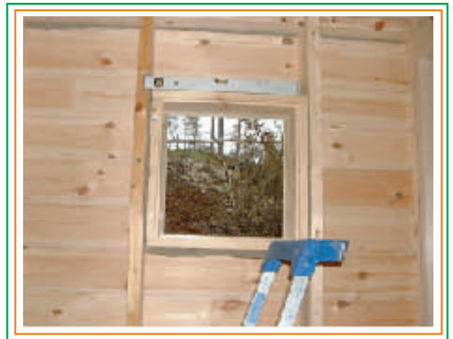
10. No top & bottom support beams are needed for small window frames.
