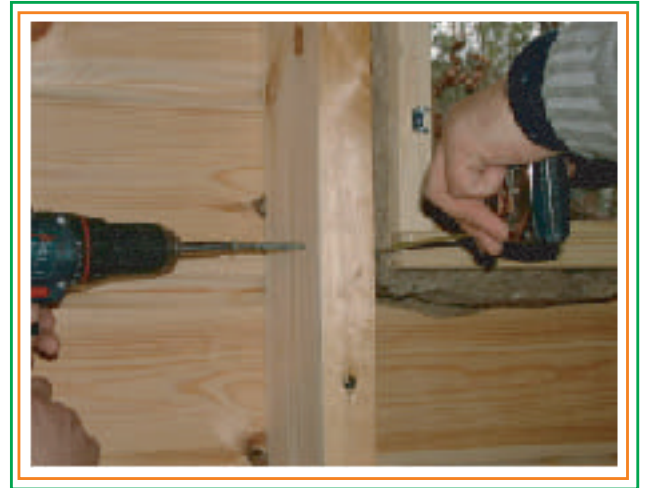
8. Small windows and ventilation shutters can be affixed with self drilling screws from the back of the post.
