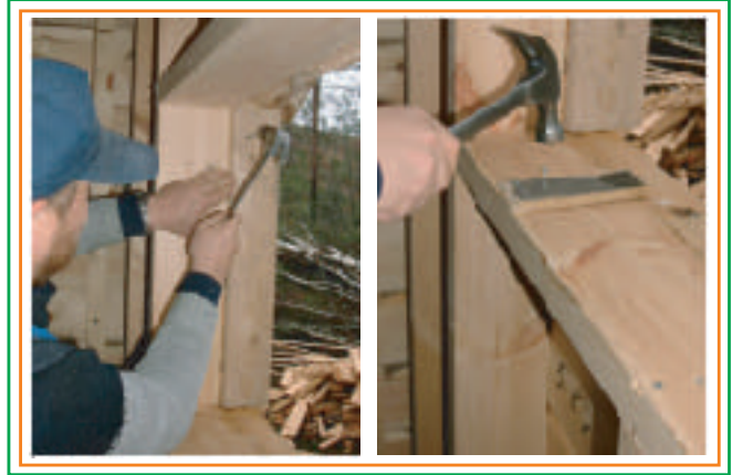
2. Install stoppers in the frame and sealing spacers on top of the lower support beam.
