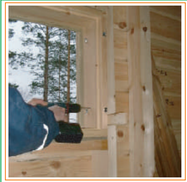
7. Screw the window frame to the wall frame.
